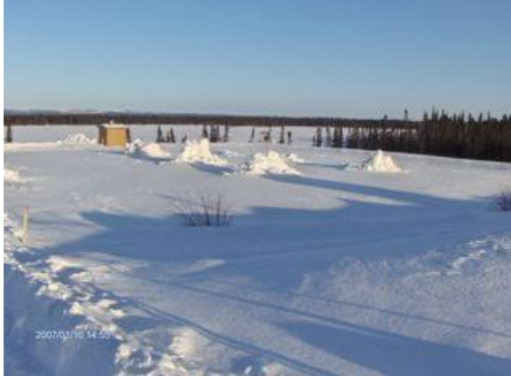
"Smokestacks" formed by air venting through lagoon ice cover
