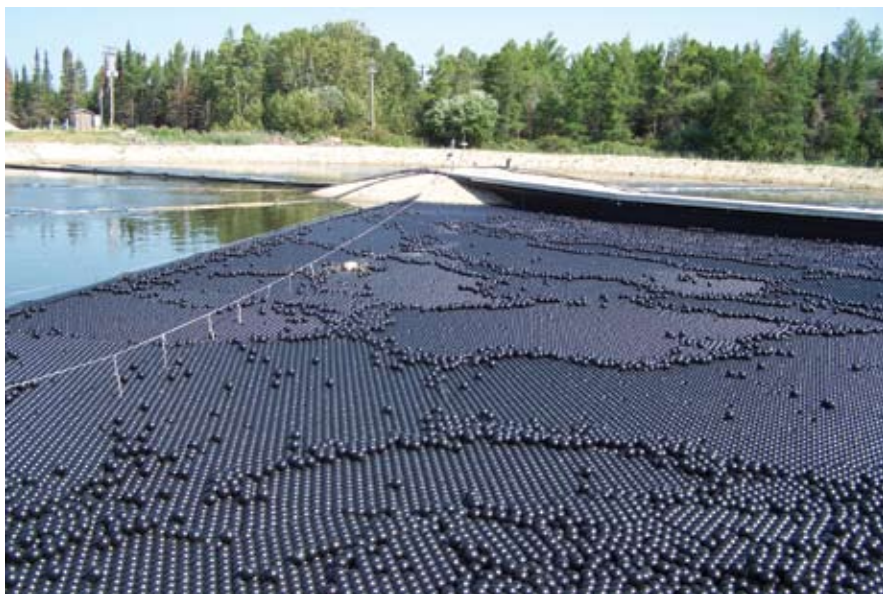
Algae control cover on setting zone.
