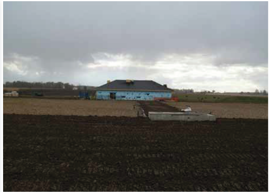
Glencoe's completed SAGR with insulating woodchips at grade.
